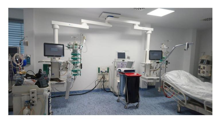
The systems can be configured as a single pendant (SINGLE) or a double pendant (TANDEM). This allows for a significant expansion of the work area while efficiently utilizing the available space. Changing work positions by swiveling the systems is easily accomplished.
